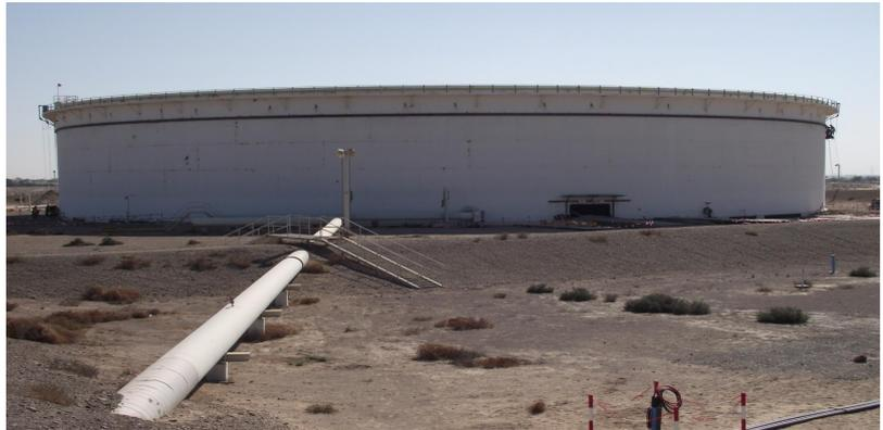
This was achieved by mechanical design substantiation of the new nozzles against the requirements of BS 2654 and relevant client standards, together with an assessment of critical defect sizes at selected weld locations at and adjacent to the new nozzles which was carried out in accordance with BS 7910.
